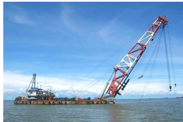
PILE DRIVING BARGE
